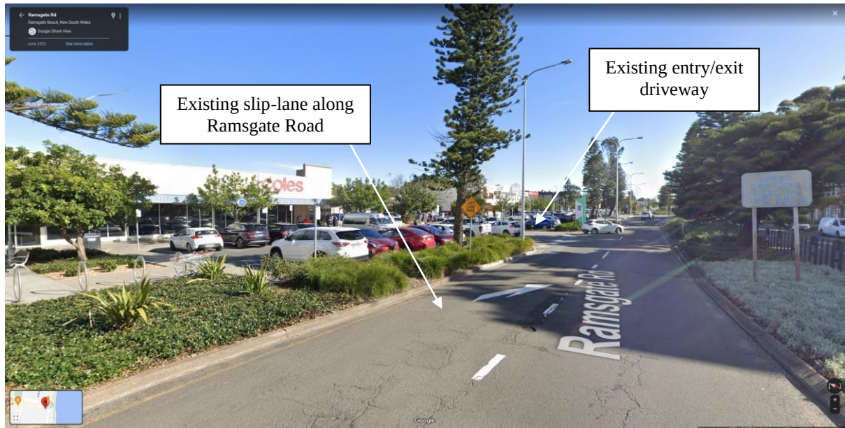
Site viewed along Ramsgate Road at the existing entry/exit driveway connecting off Council's car park
